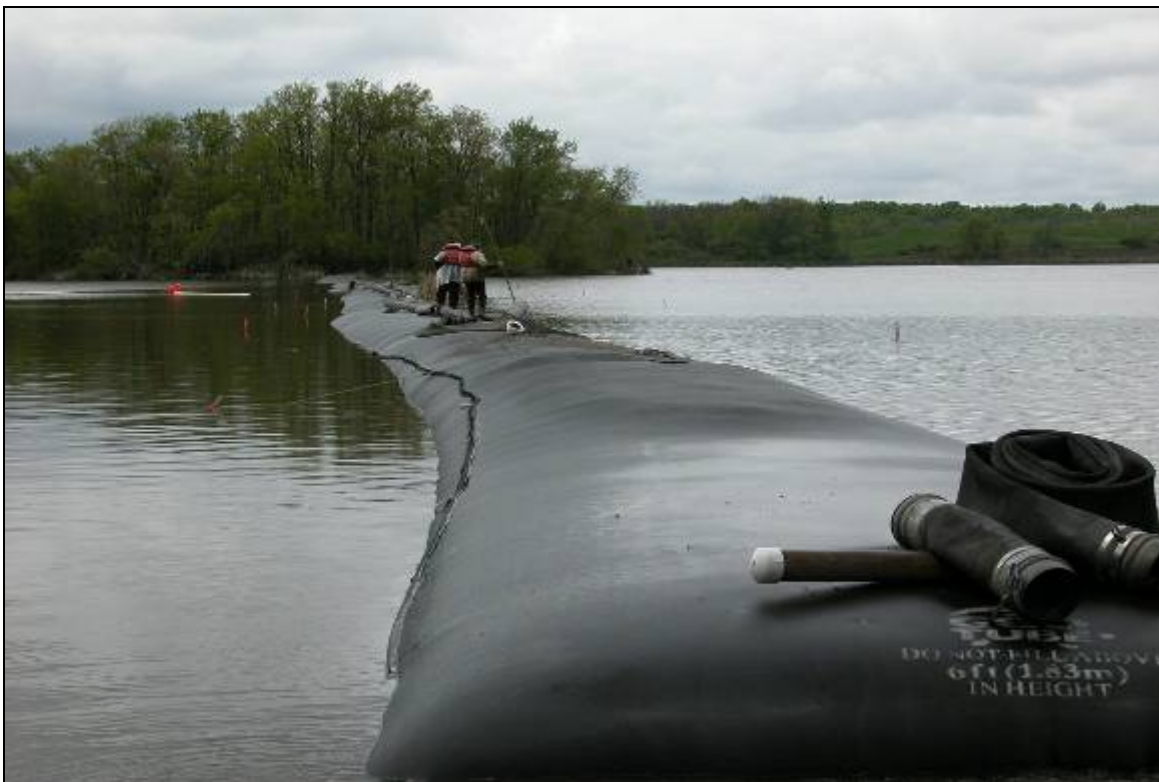
Figure 12. Geotube® geotextile containment tubes being filled with 1,500 cy of sediment. Note: This is done via hydraulic dredging from lake bottom near Wildcat Road, Lake Sinissippi, May 2006.
