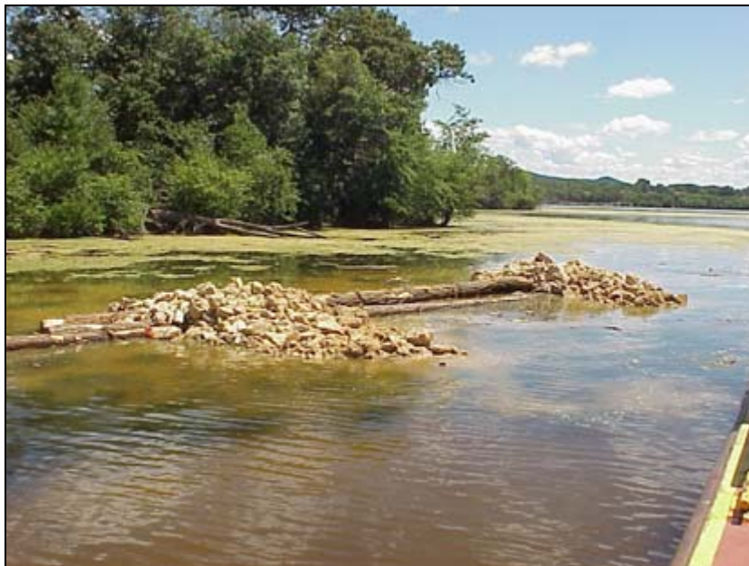
Figure 3. Rock-log Structure in Place
