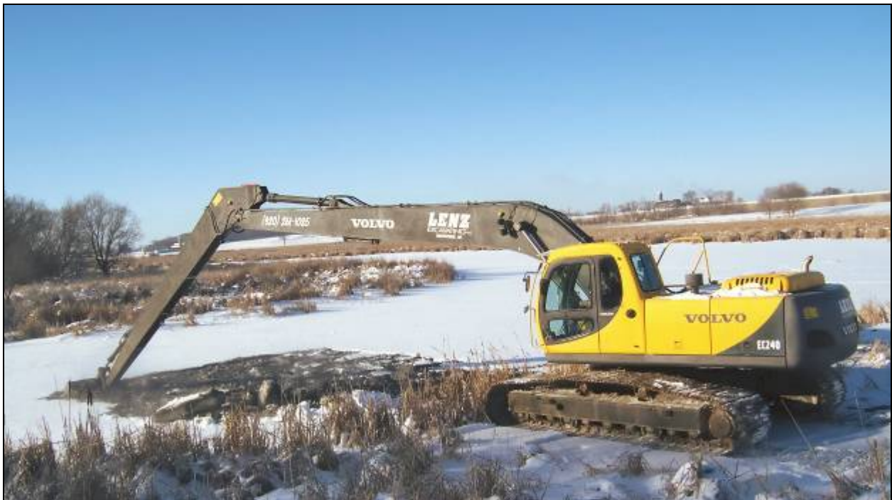
Figure 9. Mechanical dredging with long-reach backhoe at Dead Creek February 2009
