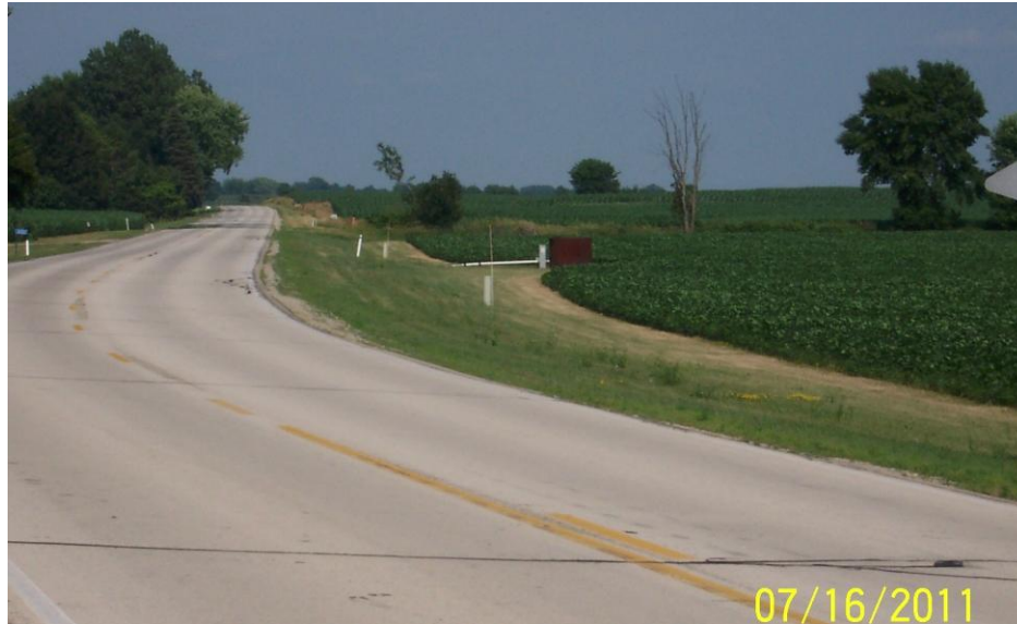
Figure 2. Field sump with drainage pump and PVC transfer pipe on the south side of Highway B, Town of Beaver Dam.
