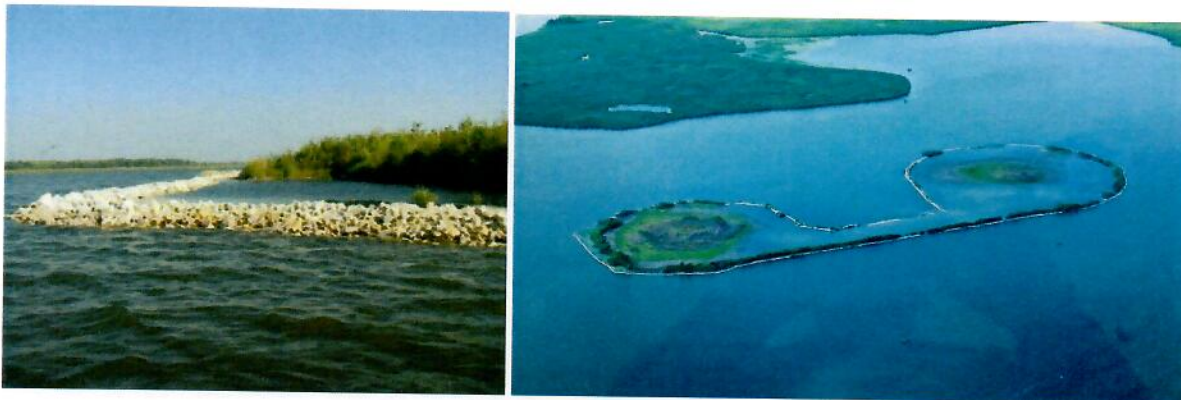
Figure B12: Artificial Island creation by the Fox Waterway Agency (IL), Grass Island, 27 acres, in Grass Lake using geotubes. The Agency is currently exploring a second island of 17 acres.
