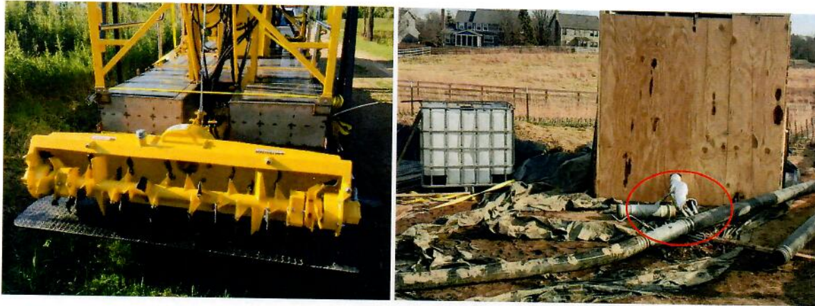
Figure B9: Cutter head dredge (left) and polymer injection (right – red oval)
